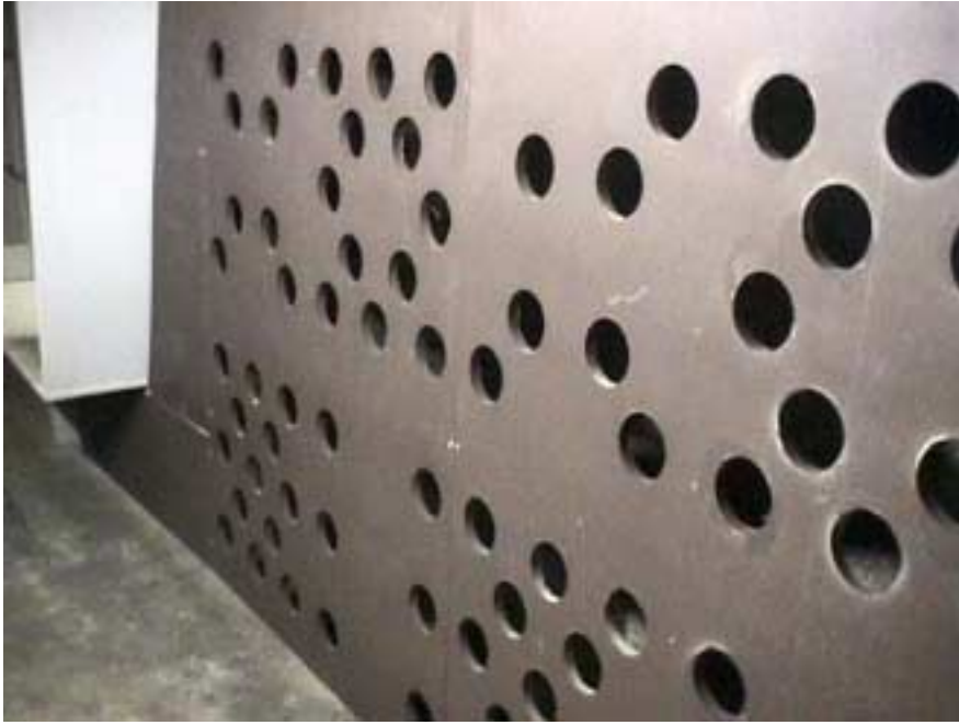
Figure 7: Helmholtz Absorber
