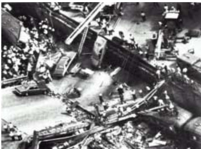
**Figure 1: Derailment and the collapse of the Bold Street bridge at Granville (NSW), 1977**
