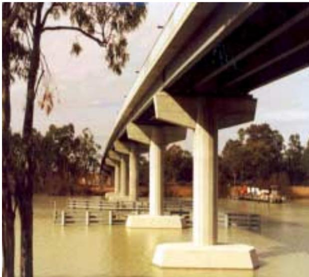
**Figure 3: Bridge over the Murray River at Berri, South Australia, 1997. First '*pier-redundant*' bridge**
