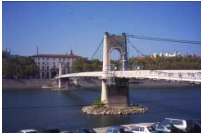
Figure 1 : The Collège footbridge in Lyon (France)
