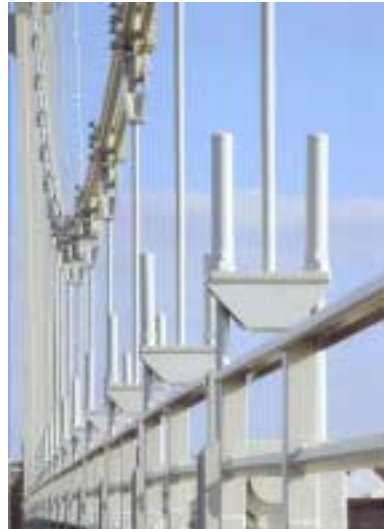
Figure 6 : the Lorois bridge : new suspension cables
