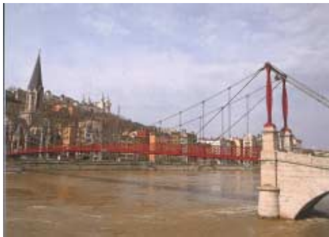
Figure 8 : Saint-Georges footbridge : general view
