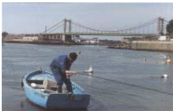
Figure 5 : General view of the Lorois bridge
