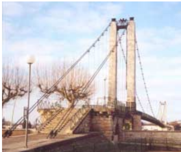
Figure 9 : the existing footbridge over the Garonne
