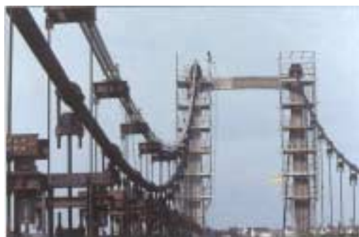
Figure 7 : the Lorois bridge : new suspension cables in place
