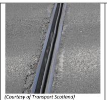
The seal is missing or sufficiently disintegrated to allow large amounts of water to flow through the joint. The seal is full of debris.
