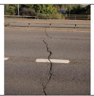
The width of the crack is greater than 25mm and the depth is similar to the depth of the surfacing. The surfacing around the crack is breaking up. There is evidence of leakage.
