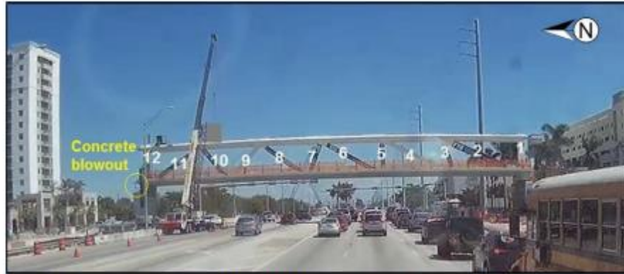
Figure 9. Still image (time stamp 13:46:43:881) from in-vehicle mounted video camera on pickup truck traveling east on SW 8th Street, showing concrete dust and debris blowout at north end (pylon pier), March 15, about 1:46 p.m.
