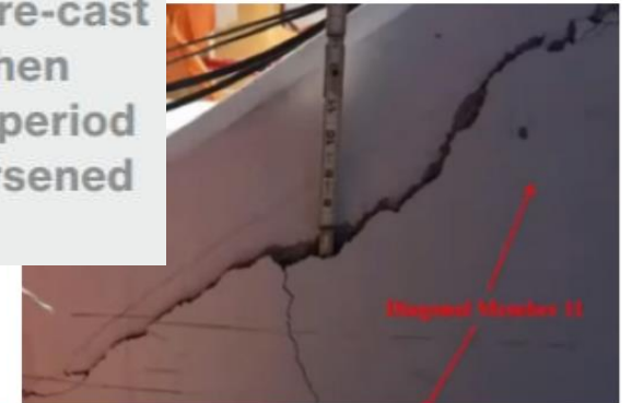
● Photo 3 Cracking to diagonal member 11 (taken from NTSB Ref 1)
