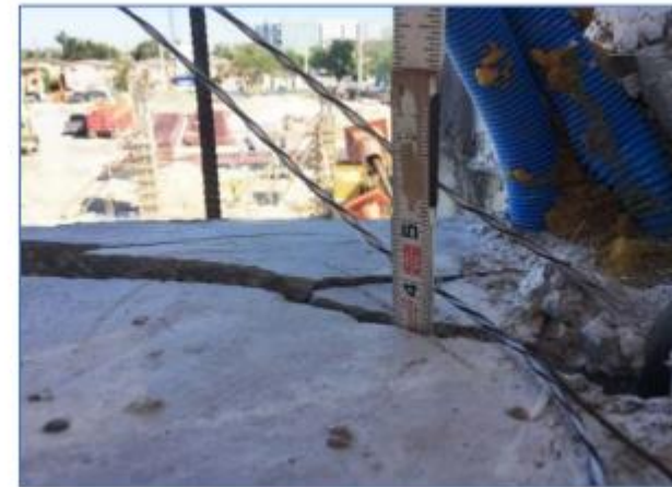
Figure 24. Cracks of 3–4 inch depth at northern end of precast main span, along west side of diaphragm 2 (north view), March 13, 11:17 a.m. (Source: MCM)
