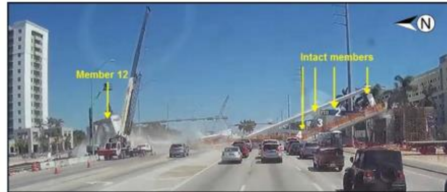
Figure 11. Still image (time stamp 13:46:44:310) from in-vehicle mounted video camera on pickup truck traveling east on SW 8th Street, showing main span completely collapsed, March 15, about 1:46 p.m.
