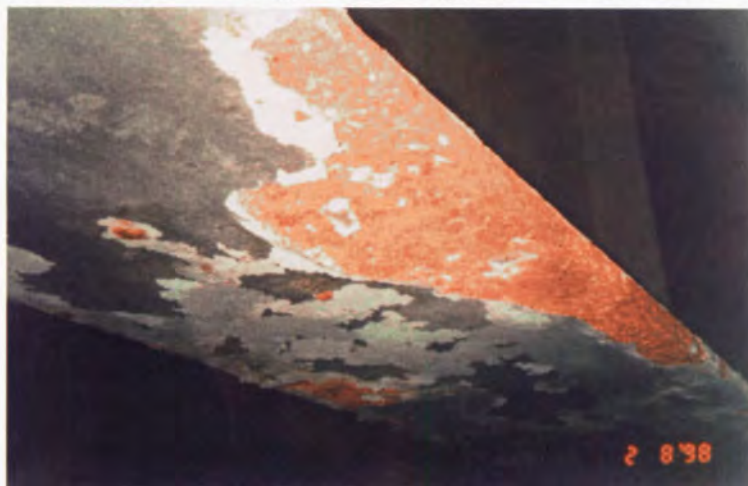
c. Severity: 3 – Flaking and missing paint on main beam
