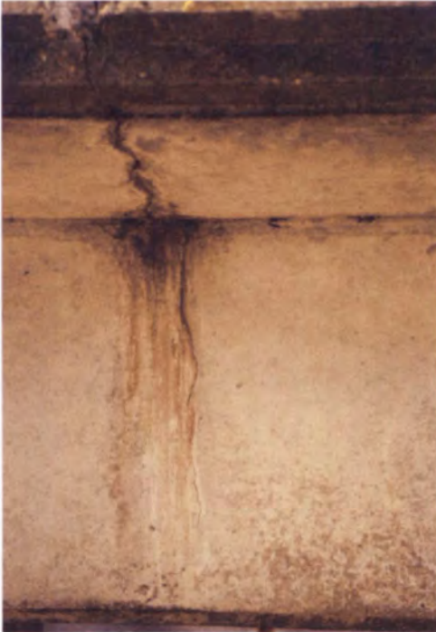
d. Severity: 3 – Significant rust staining
