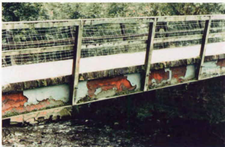
d. Severity: 4 – Breakdown of paint on footbridge beam, allowing extensive corrosion
