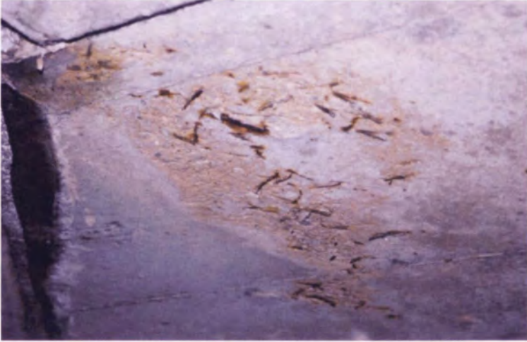
c. Severity: 2 – Rusty tie wire and debris in soffit of deck slab
