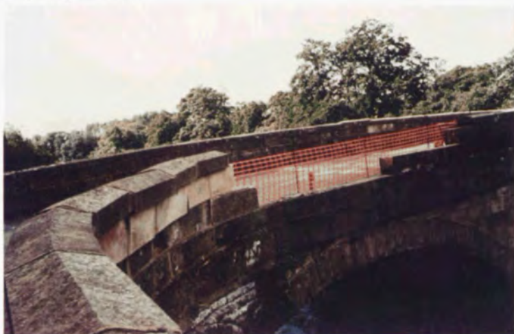
f. Severity: 5 – Impact has caused demolition of a length of parapet wall
